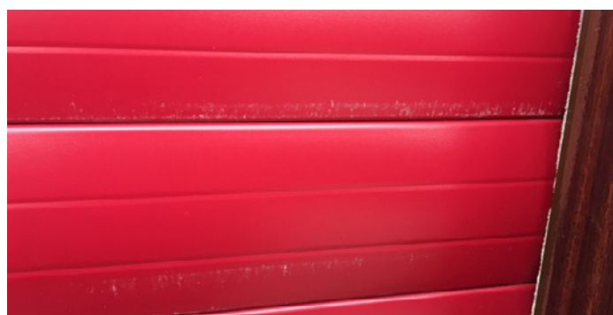
Scratches and scuffs caused by allowing grit/dirt to remain on the curtain.
