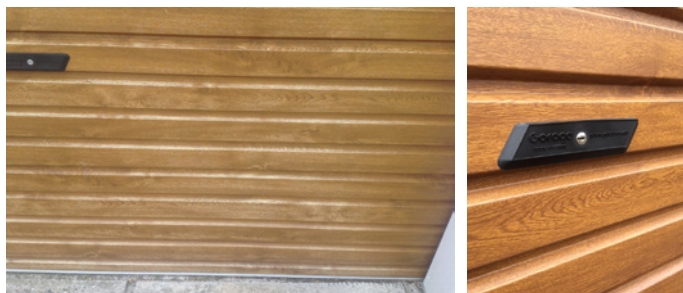
Fading due to weathering / UV radiation over time - left image compared to image of new door (right).
