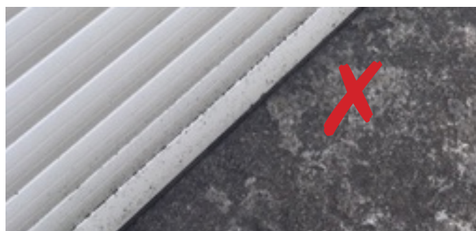
Remove dirt splashed up your door curtain after power washing driveway.
